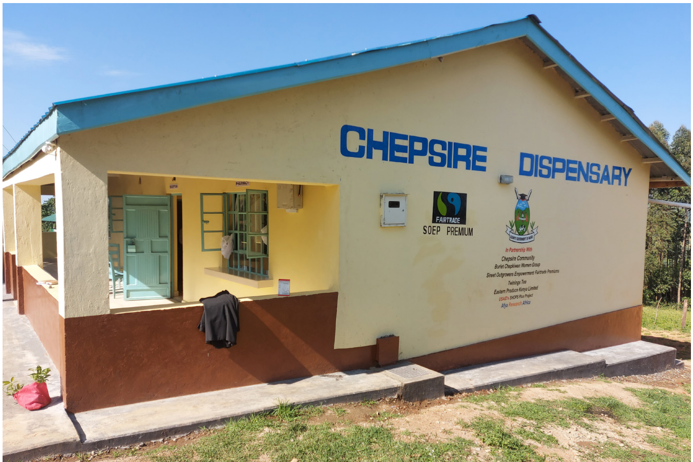
Renovated Chepsire Health Dispensary.
